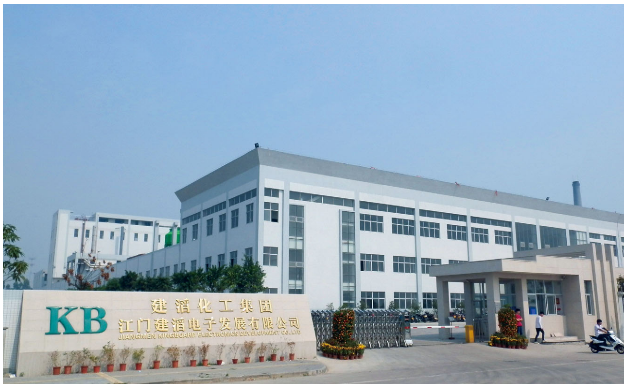
Construction work for the Jiangmen laminates plant, Guangdong province has been completed. 集團新建廣東省江門之廠房已竣工。
